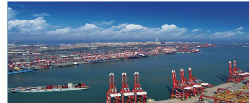
2016 the hot water reconstruction project of Qingdao port.
